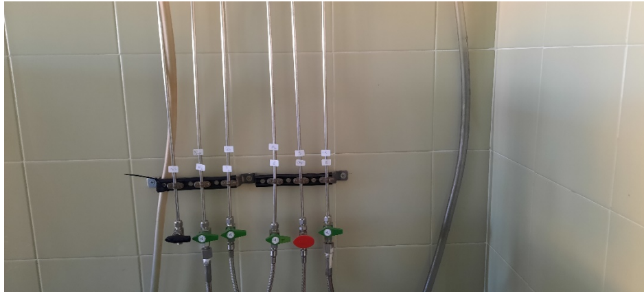
Figure 3: The valves of the bottles in the wall near to the flow meters
